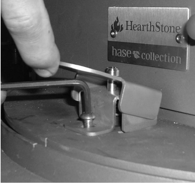
Figure 4: Remove Mounting Screw
