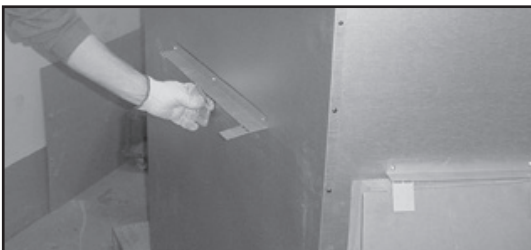
Figure 3.7 Bending Refractory Shipping Tabs Back Down
